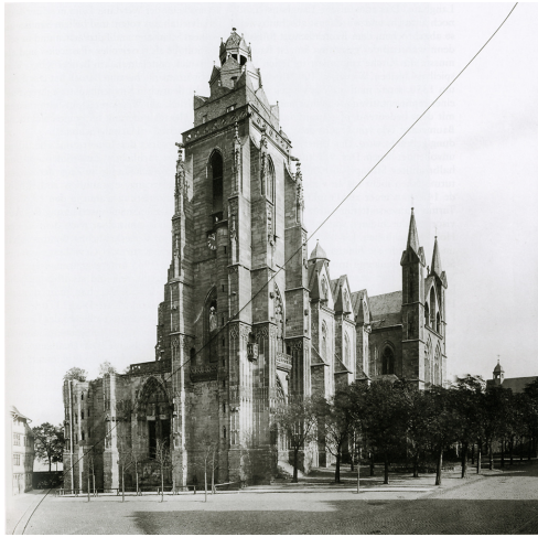
(a) Photogrammetry in the 19th century. The surveyor Albrecht Meydenbauer photographed the building with a pre-calibrated camera and could take metric measurements directly in the photo. Source: [Mey]
